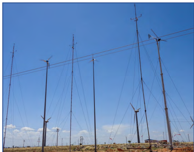
Small wind turbine testing at WTRS, Kayathar
