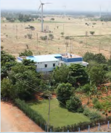
Wind Turbine Research Station
